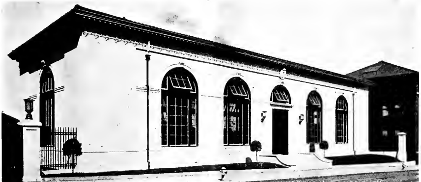
Exterior of one of the Union Iron Works' Potrero power houses.
